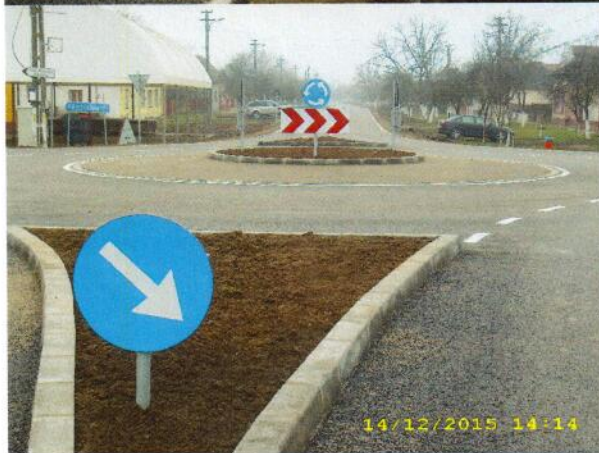
Modernizare DJ 592D Ohaba Forgaci – Racovița
